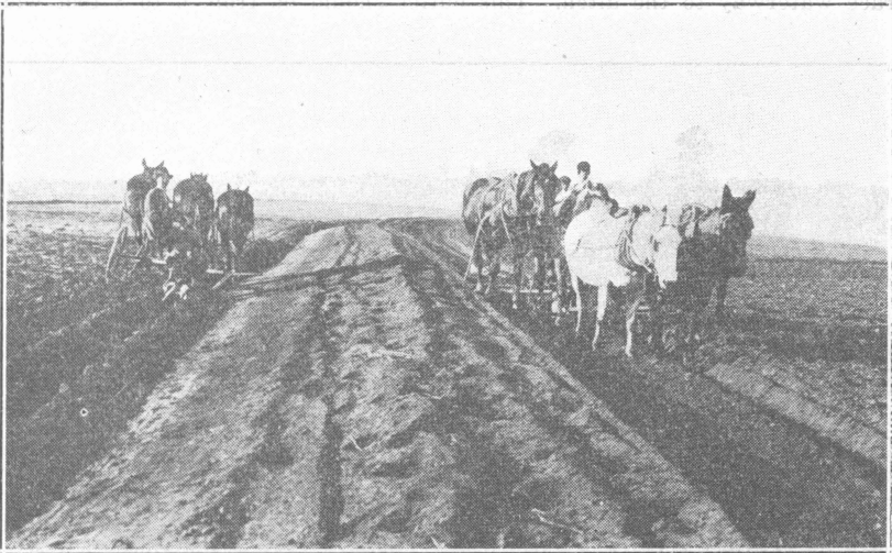
FIG. 15. Building the terrace ridge. The plow is followed by the drag.
