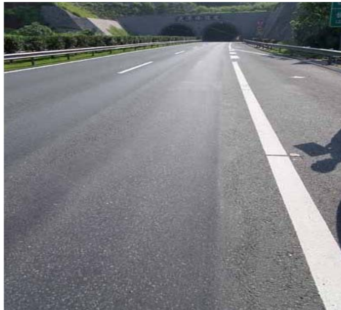
Figure 4. Permanent deformation
