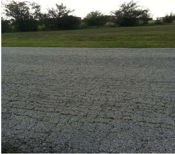
Figure 5. Fatigue cracking
