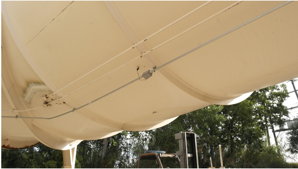
Fig. 13: Conduit along wind tunnel for wiring of circuit pressure transducers.
