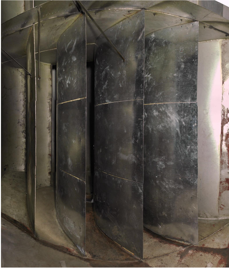
Fig. 31: Downwind view of turning vane proof of concept modifications in place.
