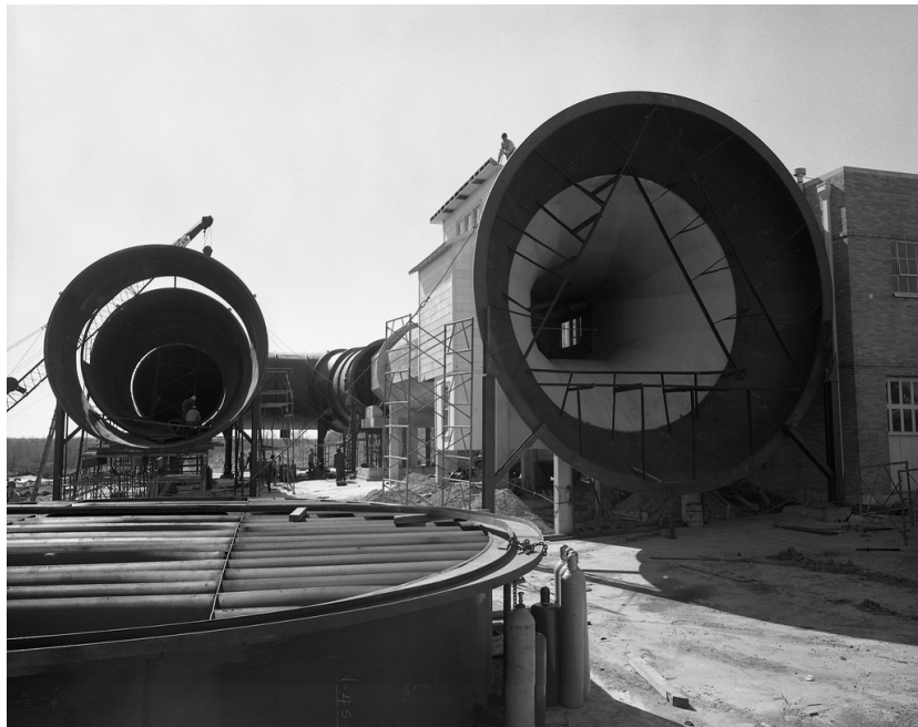
Fig. 2: Construction of the LSWT tunnel shell in 1958 to close the circuit [2].
