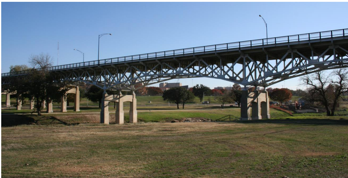
Figure 3-9. W. Lancaster Avenue over Clear Fork Trinity River.
