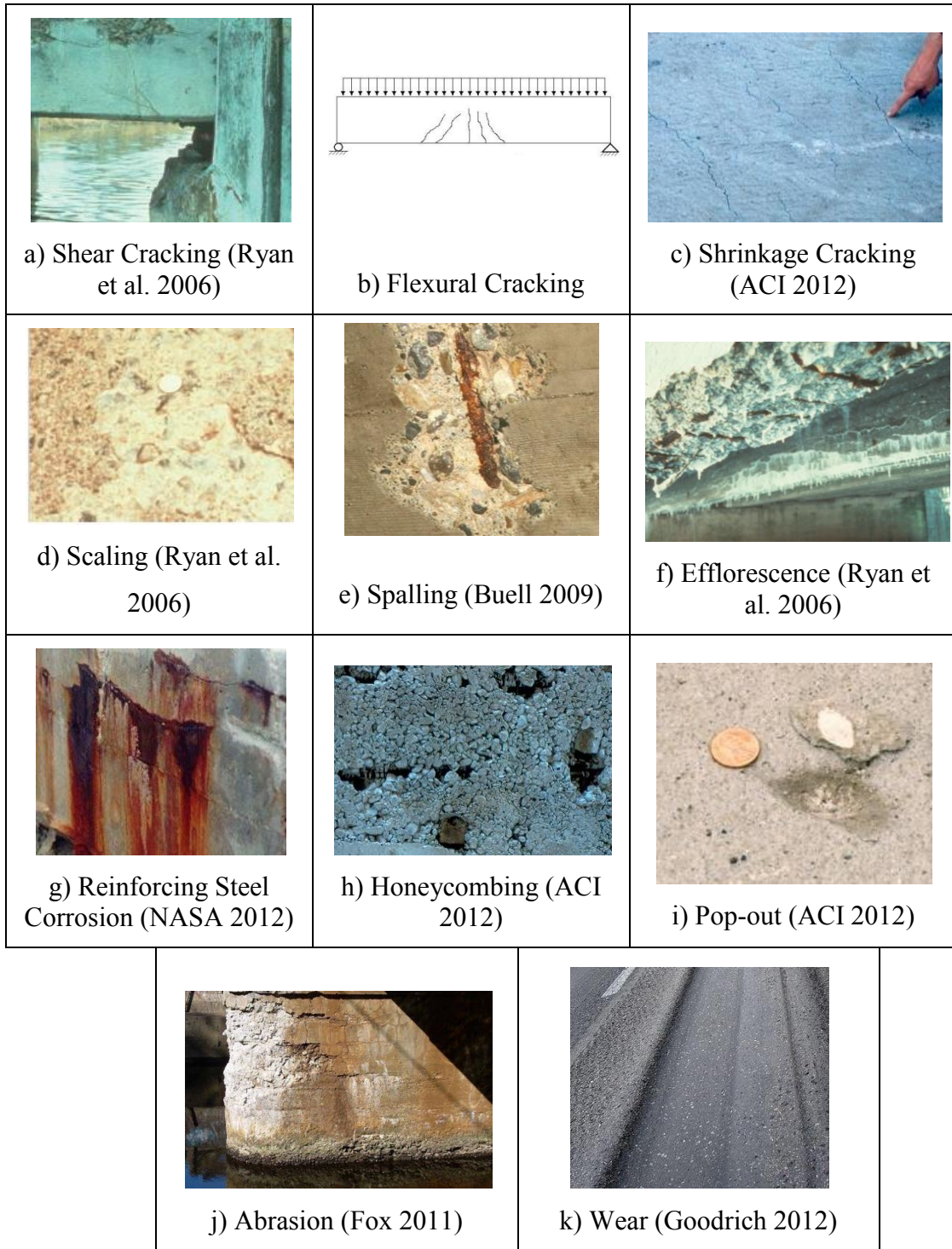
Figure 5-1. Common Defects in Concrete Elements.
