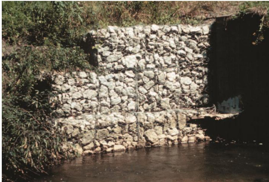
Figure 6-16. Use of Gabion to Prevent Erosion (Ryan et al. 2006).
