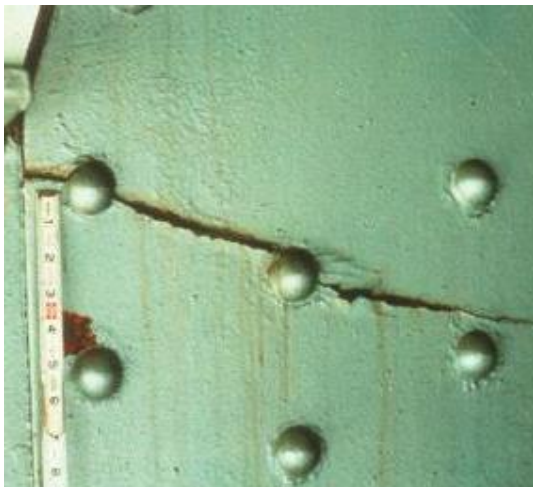
c) Fatigue Cracking (Ryan et al. 2006)
