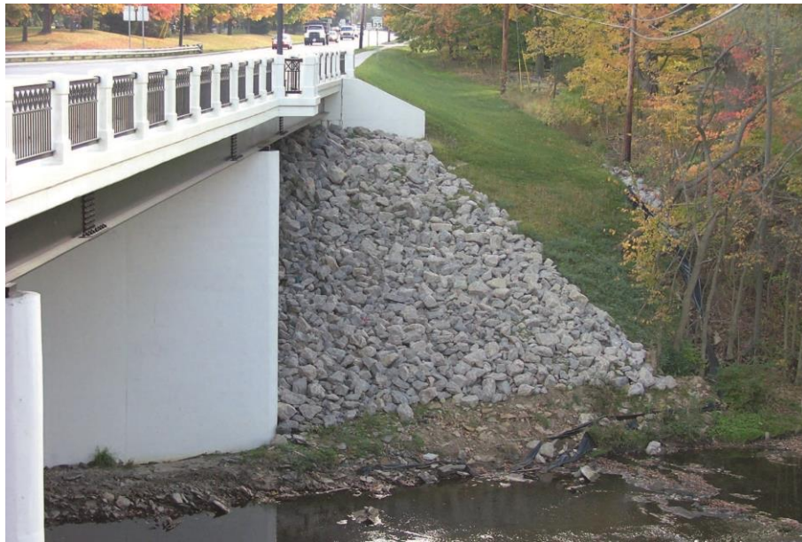
Figure 6-15. Use of Riprap to Prevent Erosion (Ryan et al. 2006).
