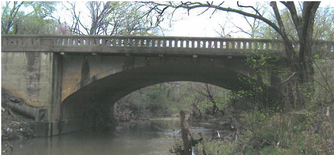
Figure 3-12. E. Vickery Boulevard over Sycamore Creek (TxDOT 2012).
