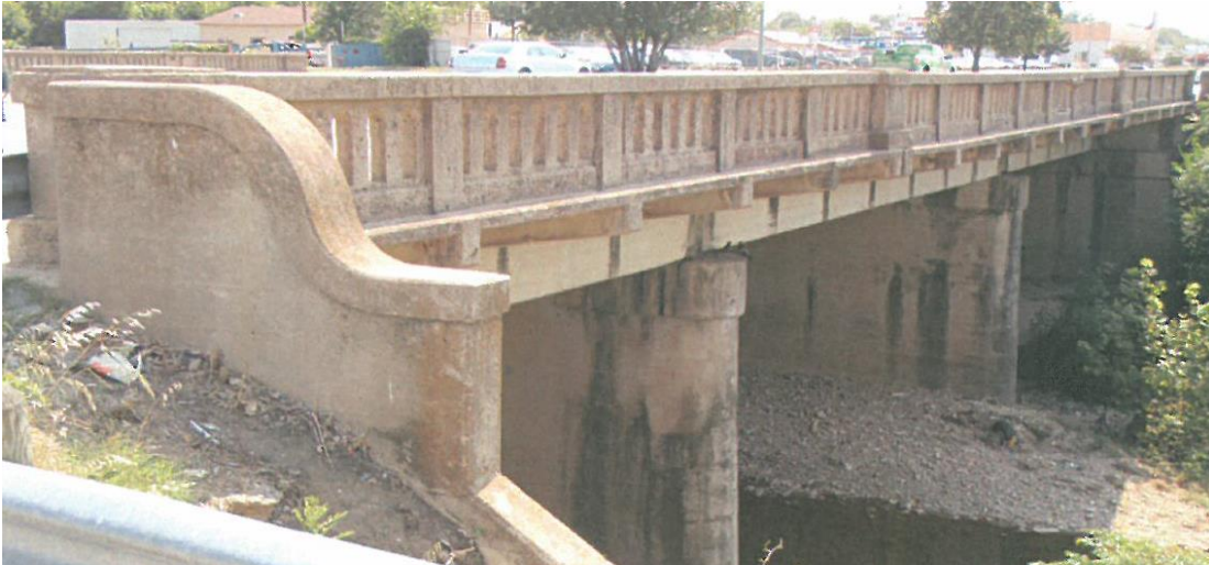
Figure 3-10. SH 180 WB over Sycamore Creek (TxDOT 2012).
