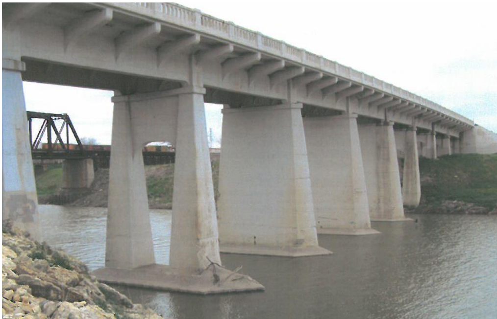
Figure 3-8. Samuels Avenue over West Fork Trinity River (TxDOT 2012).
