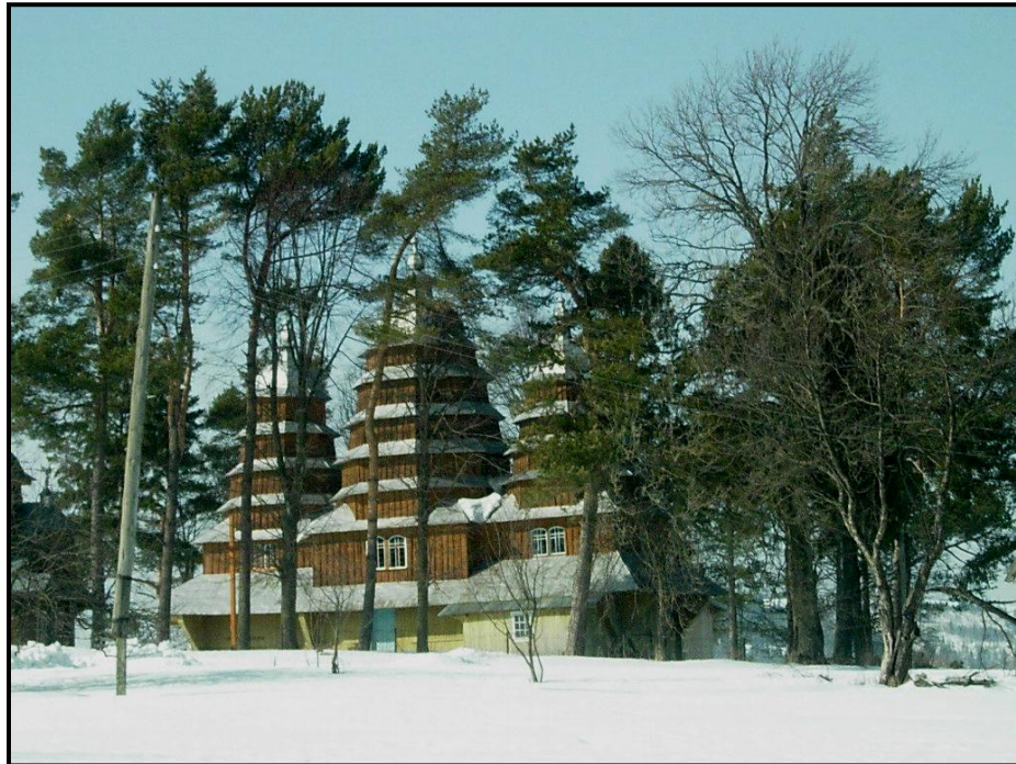
Figure 25: Exterior Picture of Church at Matkiv
