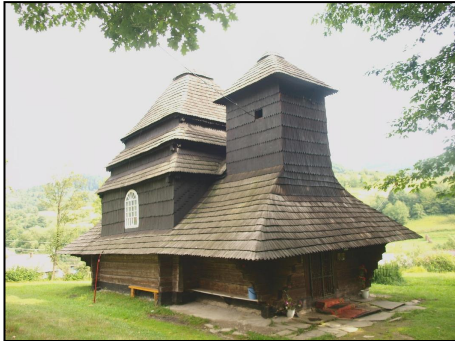
Figure 21: Close-up Exterior Picture of Church at Uzhok
