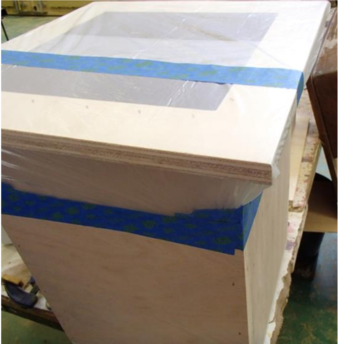
Figure 28 Taped and sealed plastic sheeting – 75 mm overlap
