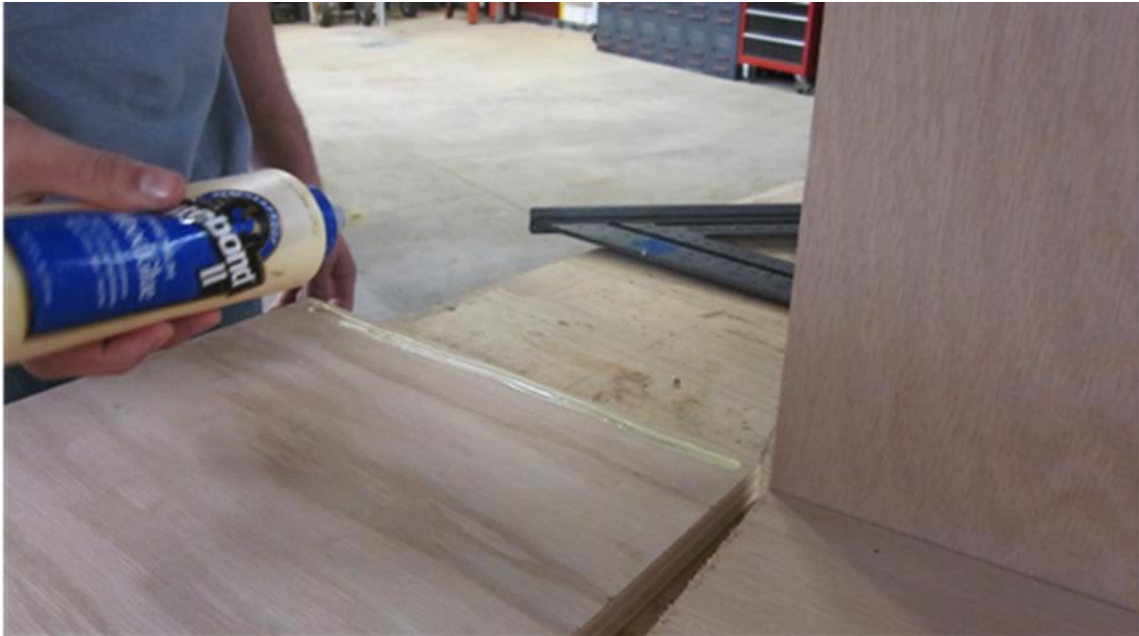
Figure 11 Gluing the edges of the box
