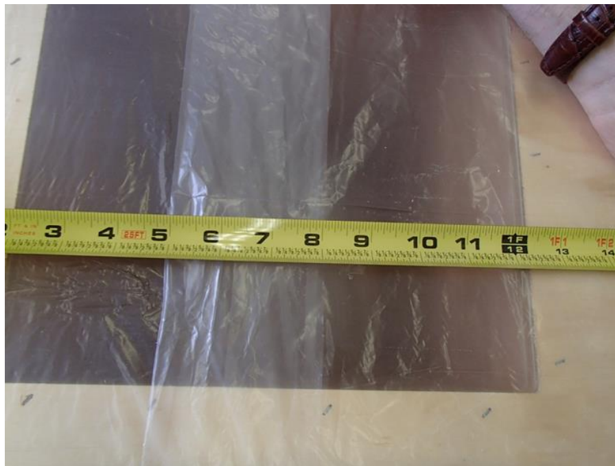
Figure 27 Placement of second plastic sheet and overlap measured
