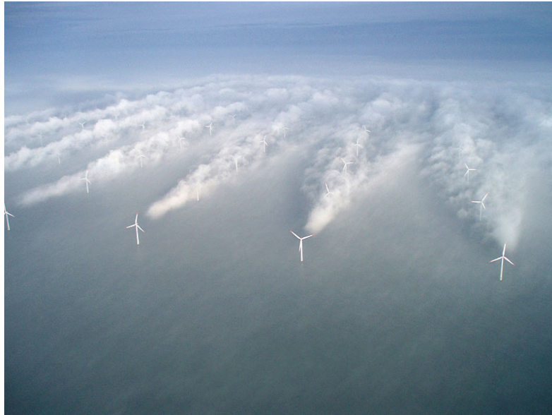
Figure 5.9 Wake turbulence behind individual wind turbines (Courtesy of Vattenfall Wind Power, Denmark)
