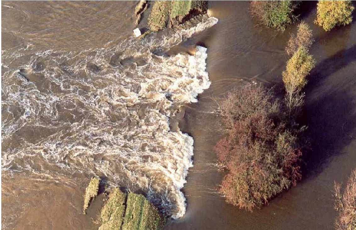
Figure 1.1. Picture depicting total failure of a levee
