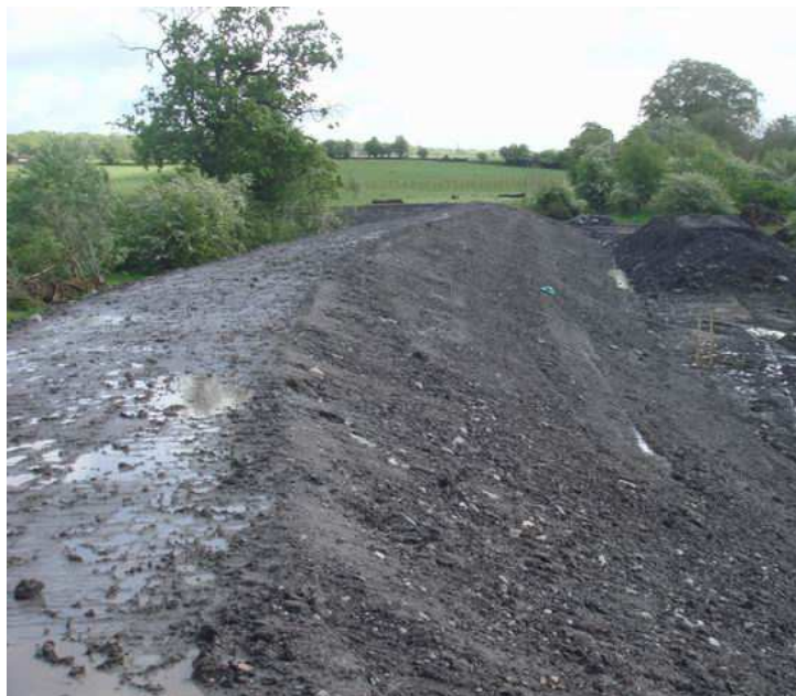
Figure 4.1. A flood protection embankment in Glaston, Scotland
