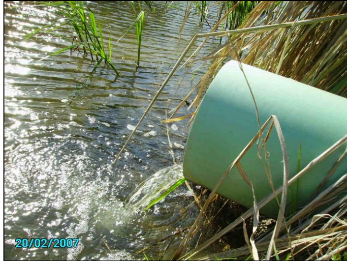
Figure 17. Outlet that received the water drain from the field during the irrigation event.
