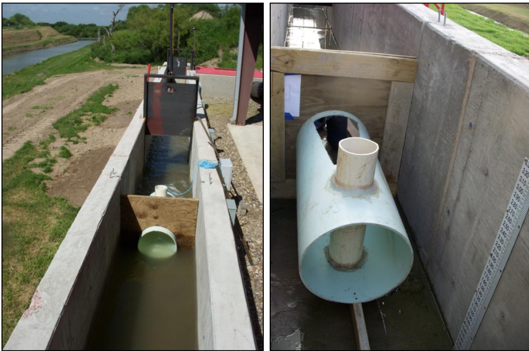
Figure 13. Calibration of the circular flow meter in the Harlingen Irrigation District.
