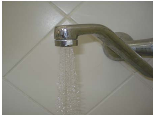
Fig. 5. Type of low-flow water tool to reduce water consumption in faucets.
