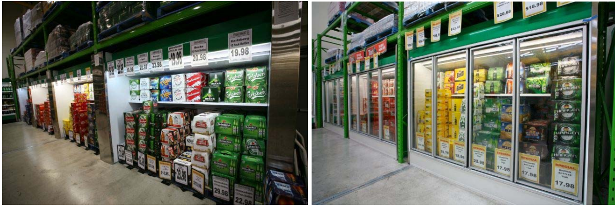
Fig. 9. Double glazed doors were retrofitted onto the beer and wine cases
