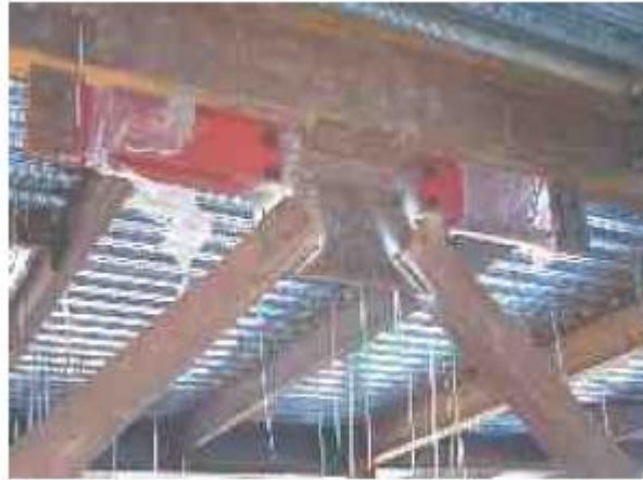
Fig. 6. Chevron-braced friction damper (Pall and Pall 2004)
