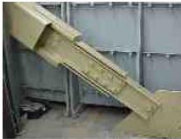
Fig. 5. Single tension/compression-braced friction damper (Pall and Pall 2004)
