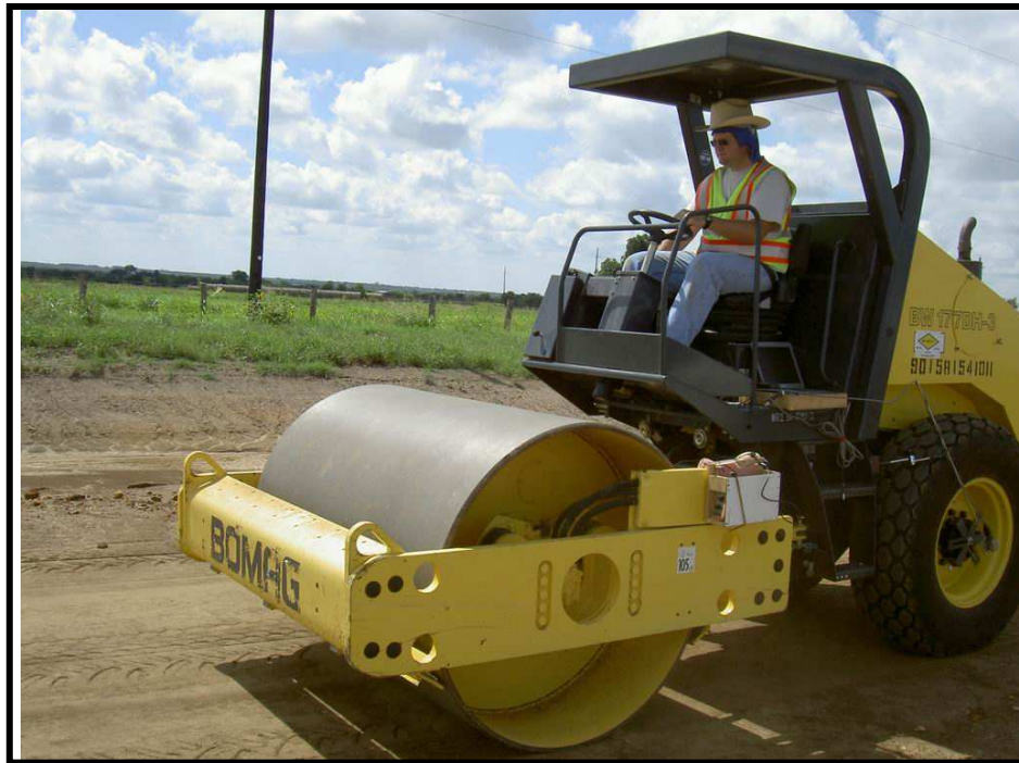
Fig. 3-1. Prototype roller system on SH 21 near Caldwell, Texas. Photograph courtesy of Dr. Wenting Liu.
