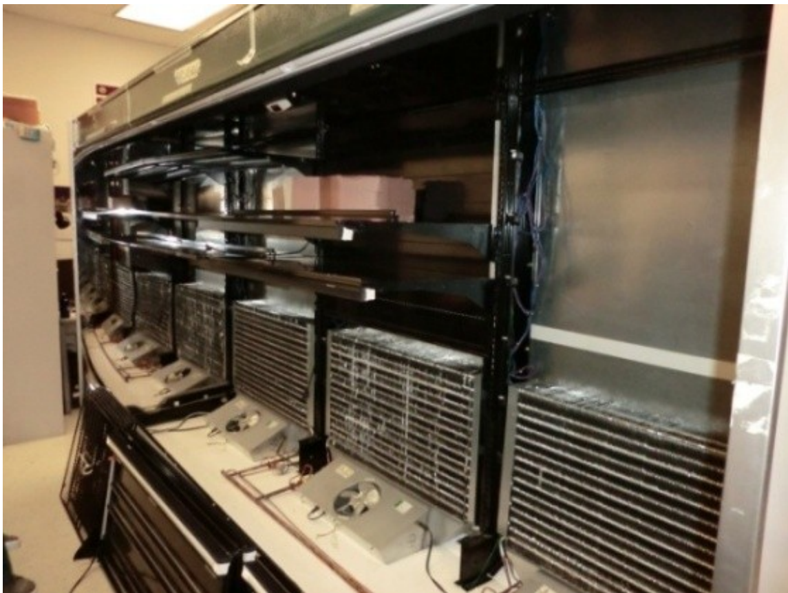
Figure 2-1 Hussmann Excel B3XC-LEP, Supermarket Open Door Display Cabinet
