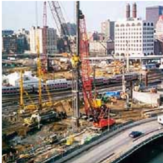
Figure 4 – 4. CA/T Project, Boston, MA (Picture from Schnabel Foundation Company, www.schnabel.com )
