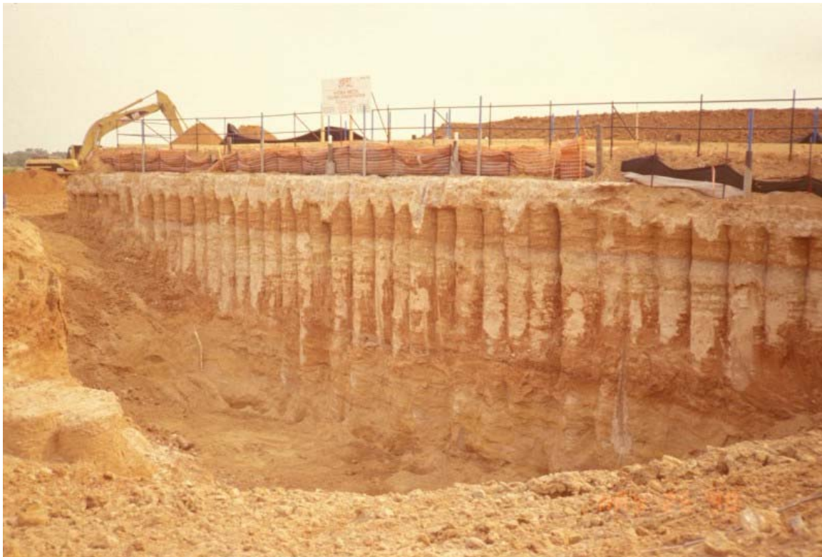
Figure 4 – 8. Completed VERT Wall (After Briaud et al., 2000)
