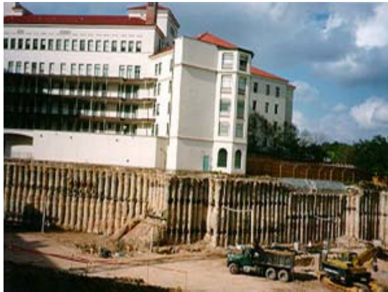
Figure 2 – 5. Hermann Hospital, Houston, TX Excavation (Picture from Schnabel Foundation Company, www.schnabel.com )
