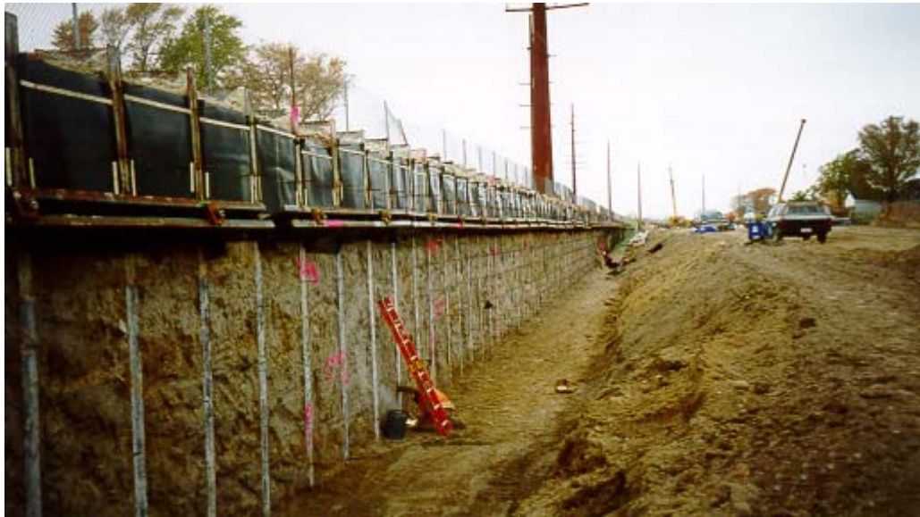
Figure 4 – 2. Lake Parkway Project (Picture from Schnabel Foundation Company, www.schnabel.com )
