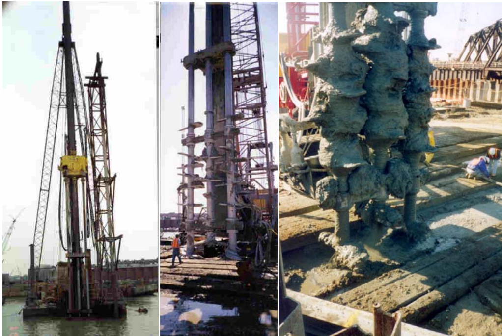
(a) M250 DMM Rig [Photos by Jakiel (2000) and McGinn]
