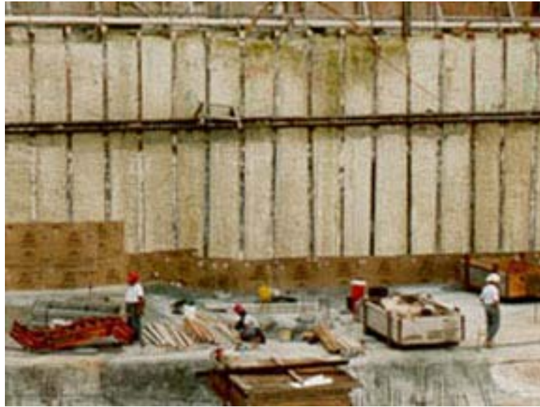
Figure 4 – 6. Marin Tower, Honolulu, HI Excavation Support System (Picture from Schnabel Foundation Company, www.schnabel.com )
