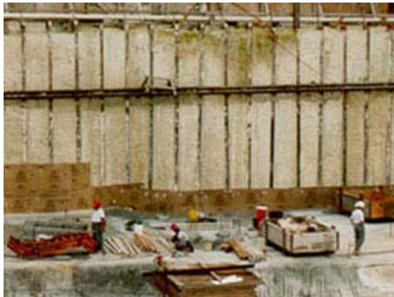
Figure 1 – 3. Marin Tower, Honolulu, HI Excavation Support System (Picture from Schnabel Foundation Company, www.schnabel.com )
