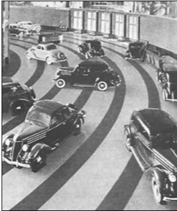
Figure 22. Linotile - 1/4 inch Thick Linoleum Tile Made for the Ford Company (after Snyder 1995:219)
