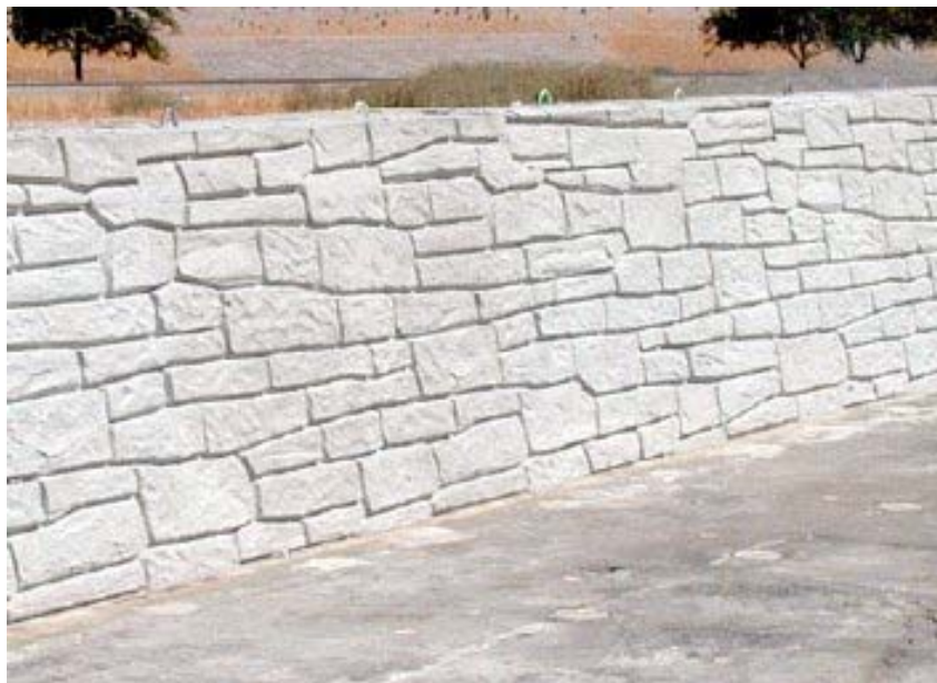
FIG. 1. Aesthetic Concrete Barrier (White et al. 2002)
