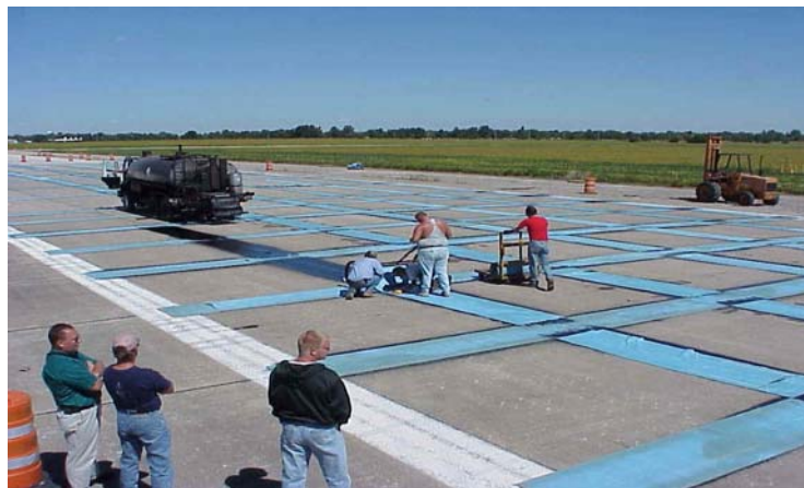
FIG. 2.18. Typical Layout of PavePrep ® Surface ( PavePrep ® Inc 2002)
