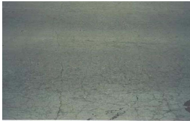
FIG. 2.9. Alkali Silica Reactivity (Visual Distress Survey Manual, SDDOT 2003)
