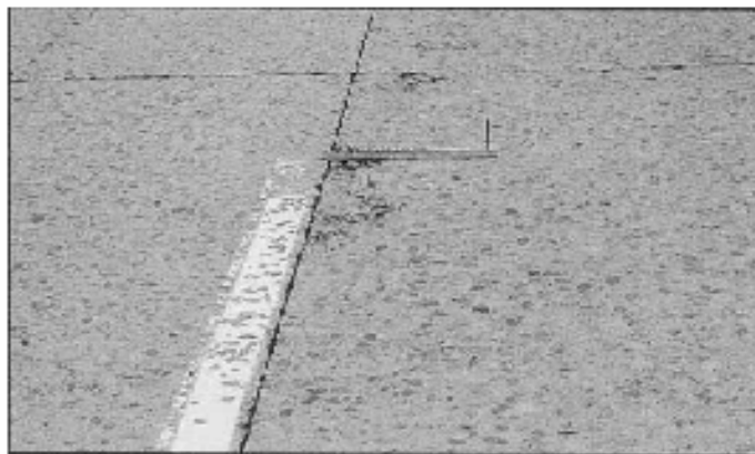
FIG. 2.1. Spalling Distress (LTPP Distress Identification Manual, FHWA 2003)
