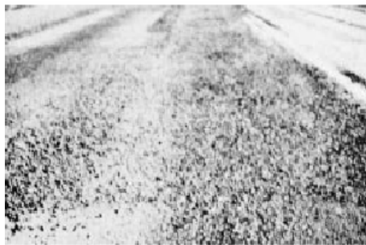
FIG. 2.14. Raveling (Iowa Design Guide, APAI 2003)
