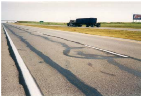
FIG. 2.16. Asphalt Overlay over Rubblized Surface (ACPA 1998)
