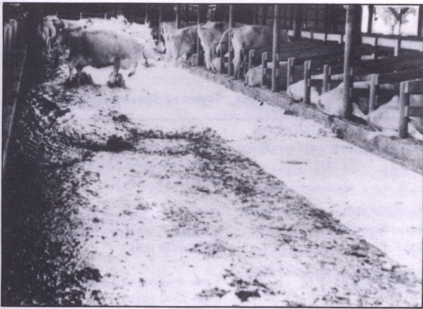
Figure 8. Flush system design should consider slope, channel length, width, water volume or flowrate, flushing frequency and surface texture.
