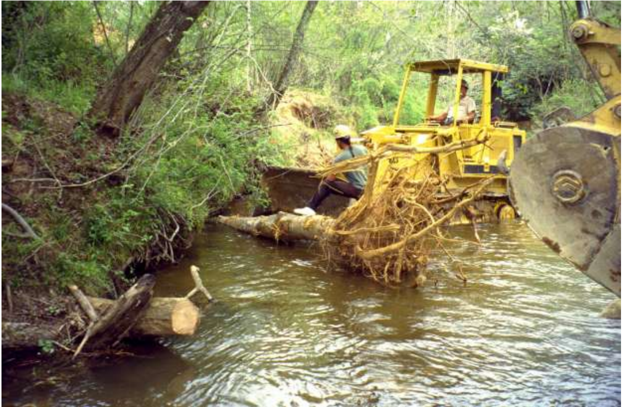
Figure 11. Installation of root wad (NCSU Water Quality Group)
