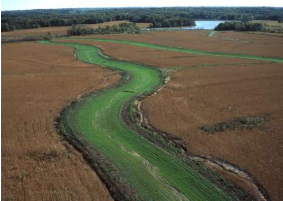
Figure 7. Grassed Waterway (Photo courtesy of USDA NRCS)
