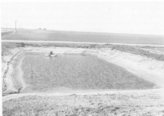
Fig. 13. A tail water recovery system showing a reservoir to collect tail water runoff and a pump to return the water to the field (USDA — Soil Conservation Service photo).
