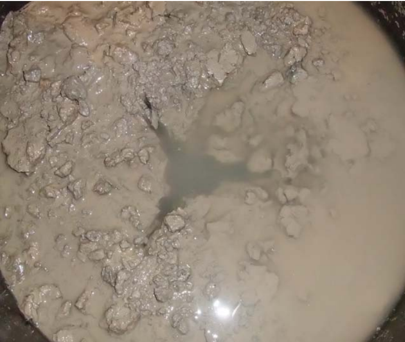
Figure 32. Typical Impact Crater After Anchor is Removed.
