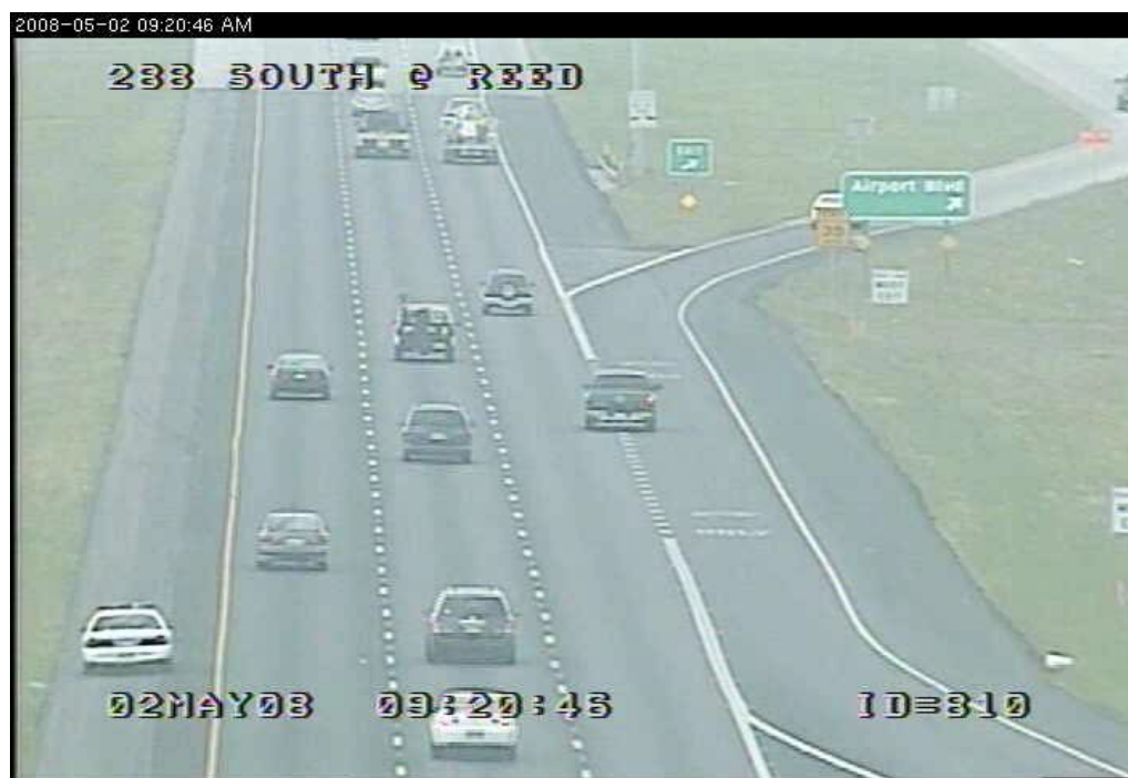
Fig. 3-1 Camera view of SH288 SB between Reed Rd and Airport Blvd
