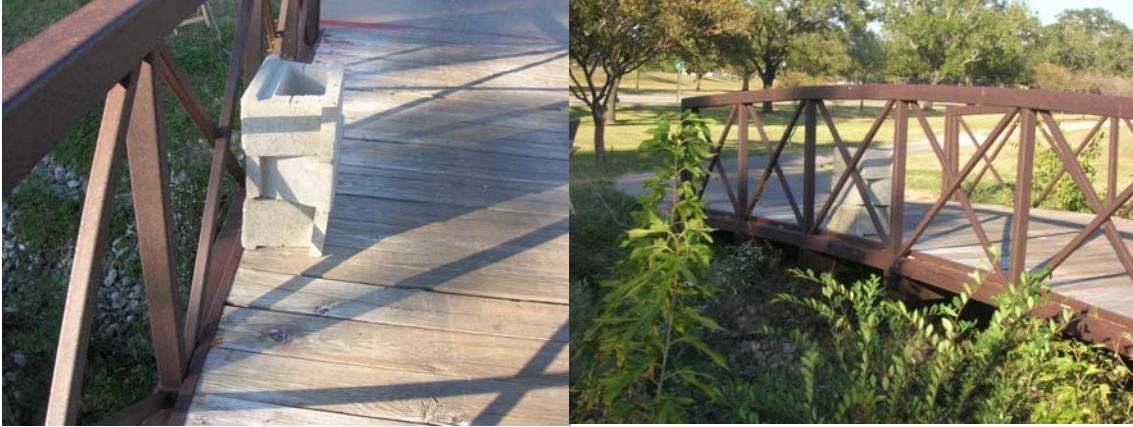
Figure 15. Added concrete blocks on the pedestrian bridge
