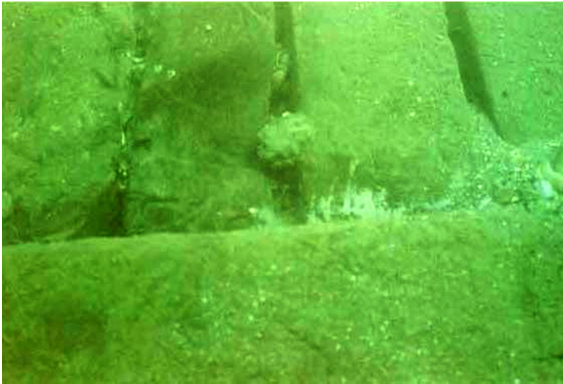
Fig. 19. Notch in adjacent timber for fastener of a toptimber. Photo: K. N. Batchvarov.
