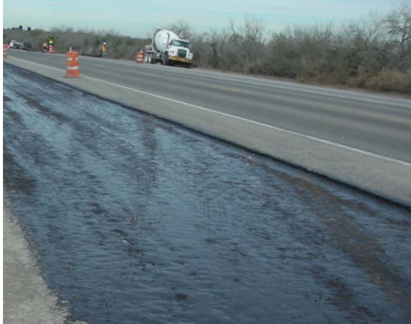
Figure 3-7. Application of Prime Coat on Flexible Base
