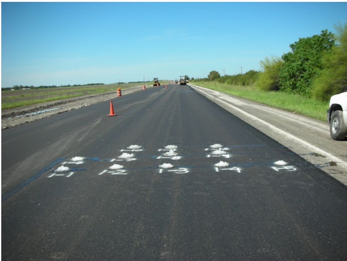
Figure 3-4. Field Coring Layout on US 87.
