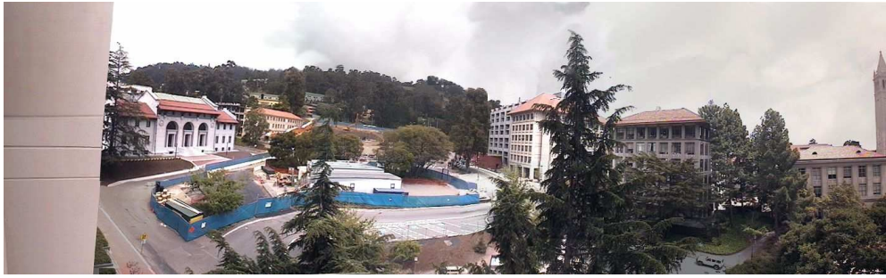
(a) Construction documentation of Stanley Hall building construction at UC Berkeley.
