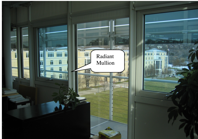
Figure 1.1 The Radiant Mullions in the IW
