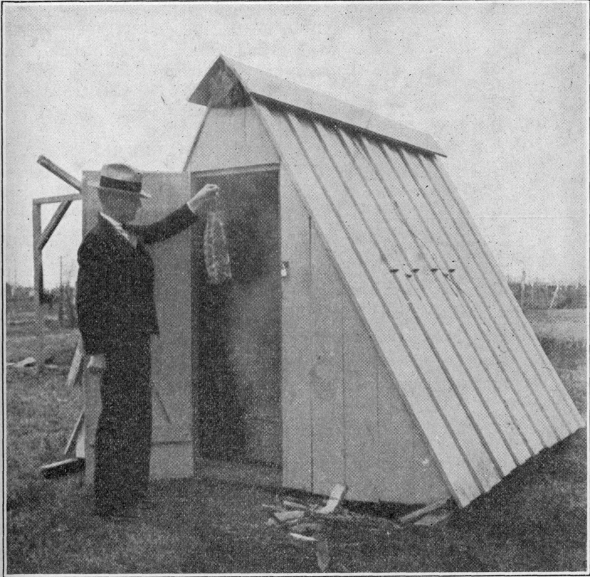
Fig. 33. A-type hog house being used to smoke meat. The fire can be built in an ordinary galvanized tub which has been partially filled with dirt. The tub should be partly covered with a piece of sheet iron to deflect the heat away from the meat.
