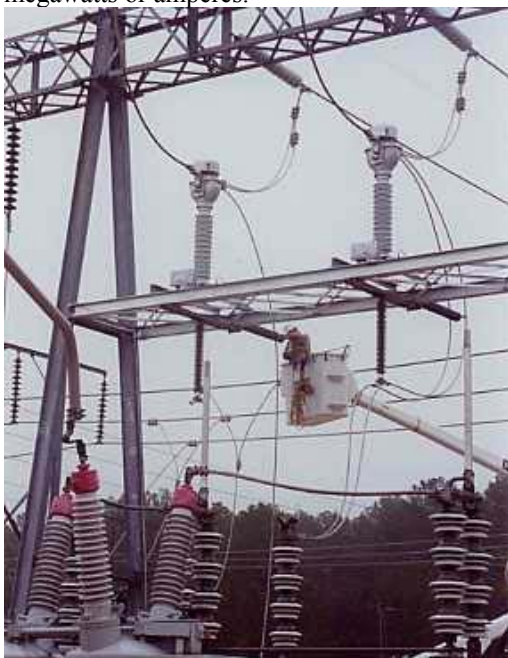
Figure 1. LCRA Transmission Construction crew installing an optical current transformer on overhead 138KV lines at a Sim Gideon Generator.
