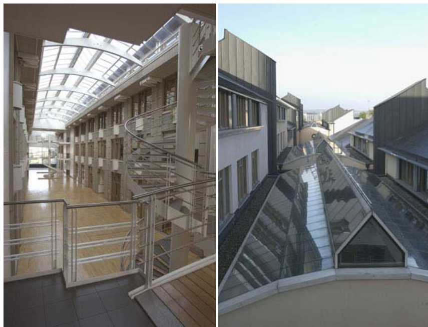
fig. 3 Views of the atrium (03_3161 and 03_3166 © MET D434)
