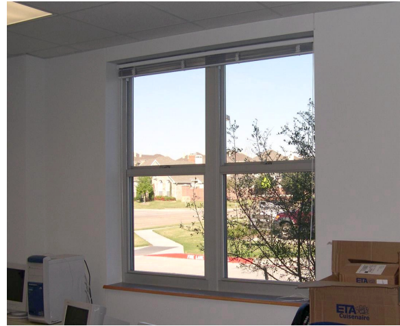
Figure 2. Photo looking out classroom 319 window
