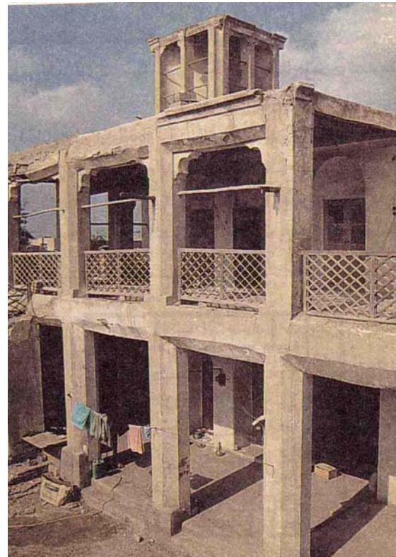
Figure 5- Shenasil is a local portico that shades the windows and walls of building. Many of outdoor activities are carried out in this space.
