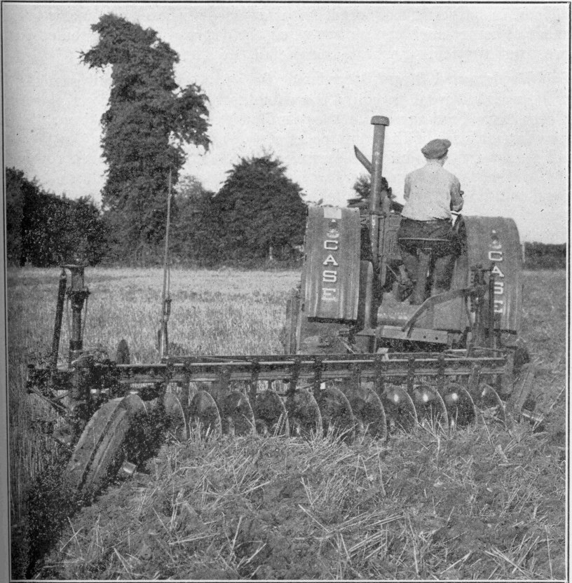
Figure 5.—The combine has brought about the development of a new plow known generally as the one-way disc plow. It is capable of cutting a strip 10 feet wide to a maximum depth of 7 inches. 20 to 30 acres can be plowed in a day with an outfit of this kind.
