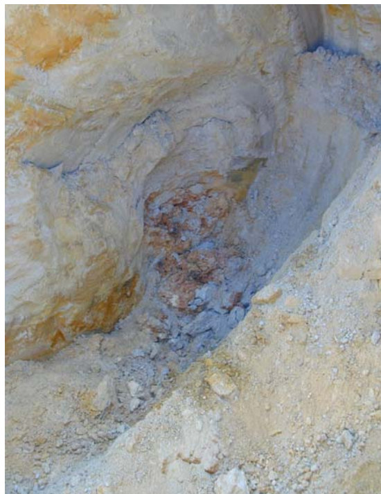
Fig. 29. A tunnel found at Malakoff in sinkhole S-5 during reclamation. The tunnel was filled with oxidized sand
