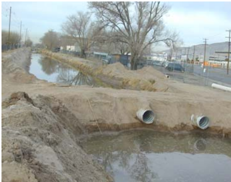
Picture 2: Ponding test site 2
