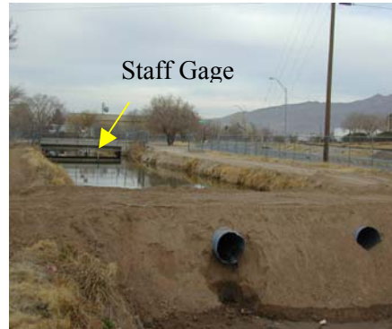
Picture 3: Ponding test site 3
