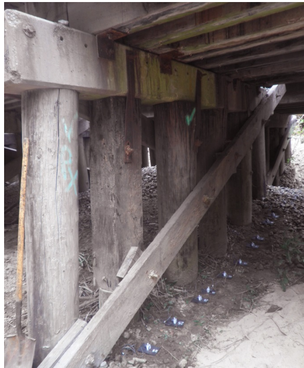
Figure 2.34: String Potentiometers Under Span 9 of Bridge 816.9
