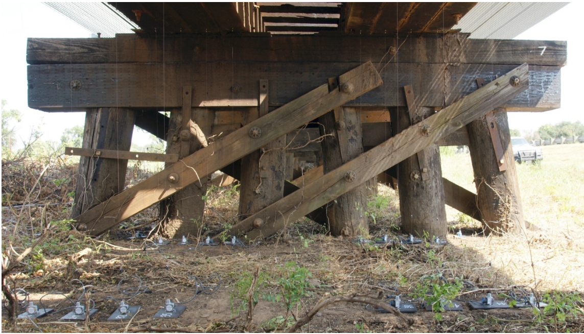
Figure 2.25: String Potentiometers Under Span 7 of Bridge 17.14
