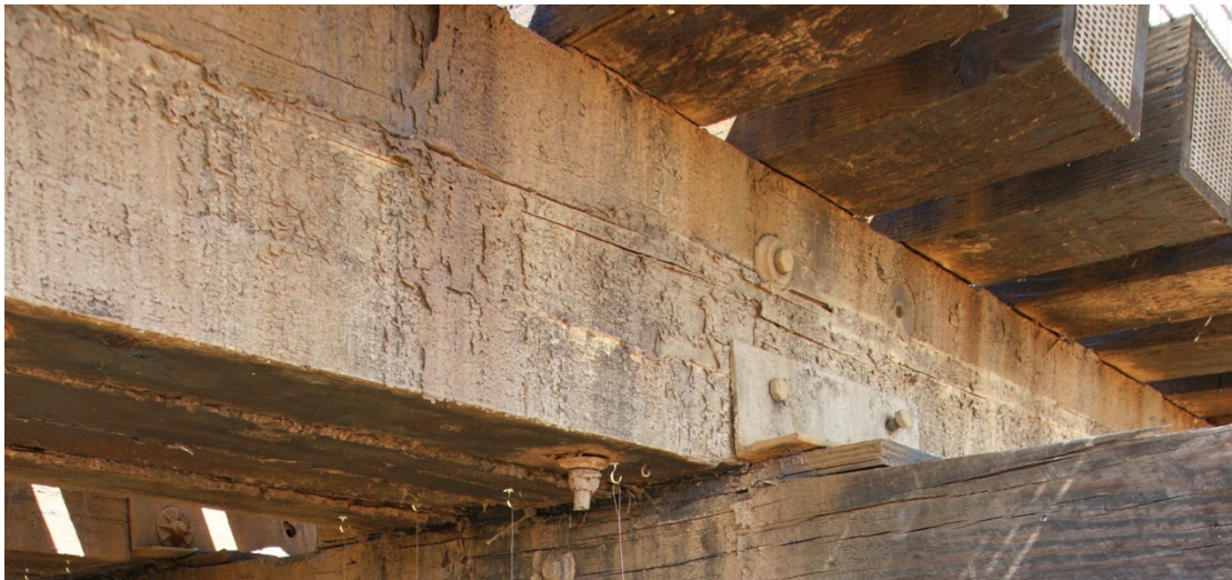
Figure 2.21: Bridge 17.14 Stringer Detail
