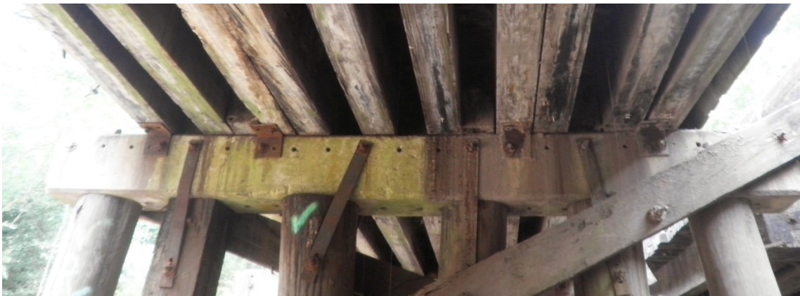
Figure 2.30: Bridge 816.9 Bent-Cap and Stringer Detail
