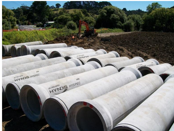
Figure 3. Rubber Ring Jointed Drainage Pipe
