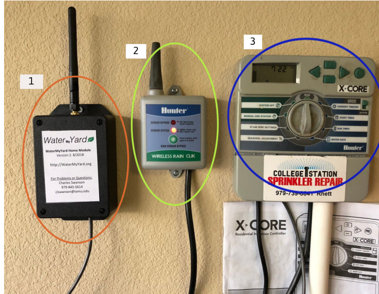
Figure 3.5: The WMY module post-installation (1) at homeowner’s residence. The module can function as a solitary add-on to the irrigation controller (2) or in tandem with a rain sensor (3)
