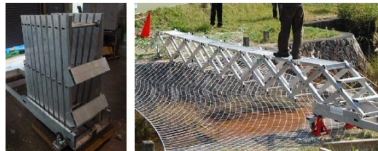
Figure 2.37 Emergency bridge in folded and deployed configurations [73, 74].
