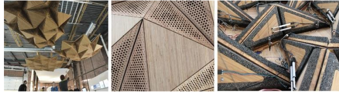
Figure 2.12 (left) Resonant chamber installation, (center) Magnified panel view, (right) Actuators and wiring system behind panels [38].
