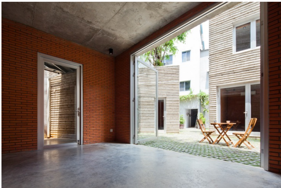
Figure 4.8. View of the interior space of box01 looking towards the courtyard, box03 , and box04 . Note the use of brick on the interior walls and polish concrete for the floor. Photograph provided by VTN Architects (H. K. T. Nguyen, personal communication, May 19, 2016).
