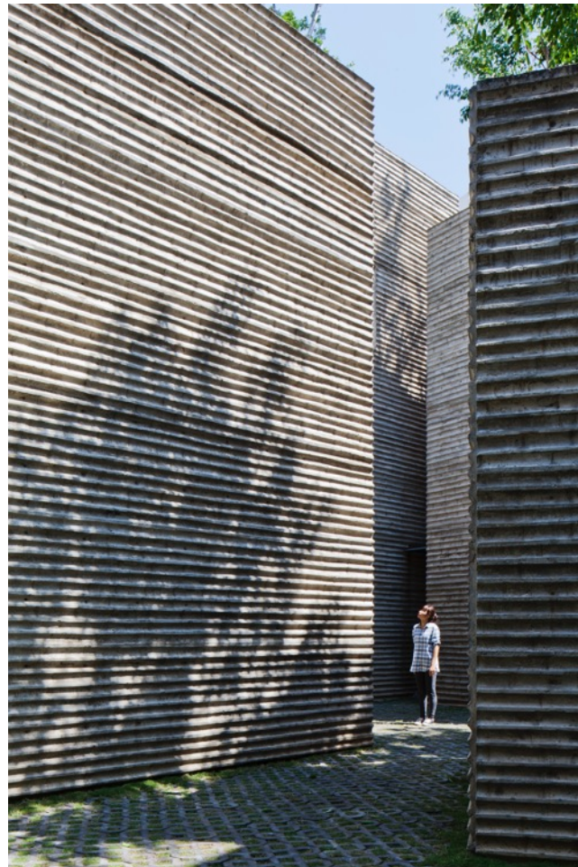
Figure 4.6. Detail of the fluted concrete exterior walls. Photograph provided by VTN Architects (H. K. T. Nguyen, personal communication, May 19, 2016).
