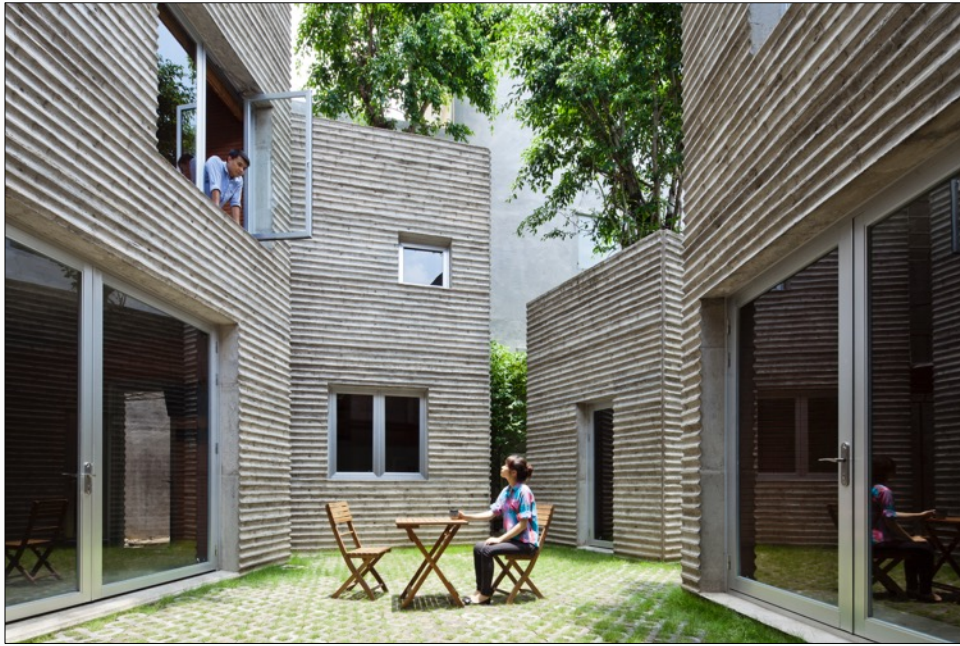
Figure 4.34. All fenestrations in the HFT use maximum area of transparency. Photograph provided by VTN Architects (H. K. T. Nguyen, personal communication, May 19, 2016).
