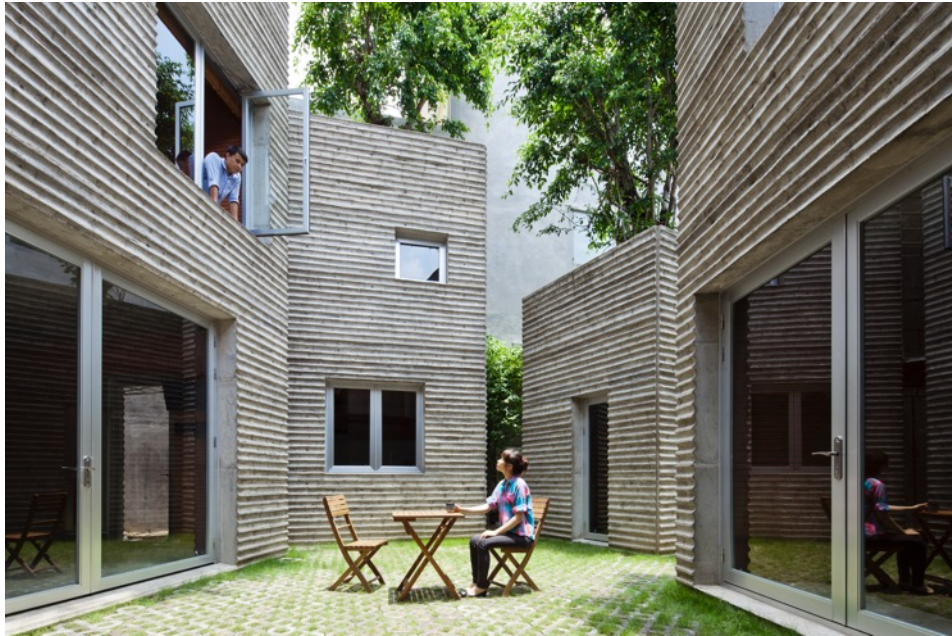
Figure 4.7. Another view of the fluted concrete exterior walls. Also note the use of grass tile cement bricks. Photograph provided by VTN Architects (H. K. T. Nguyen, personal communication, May 19, 2016).
