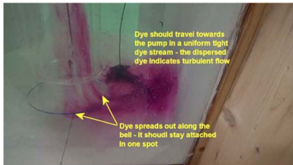
Photo 5-1 Unsteady Flow Around the Pump
