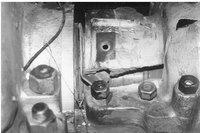
Figure 7. Turbine Inboard Bearing Cap Split.
