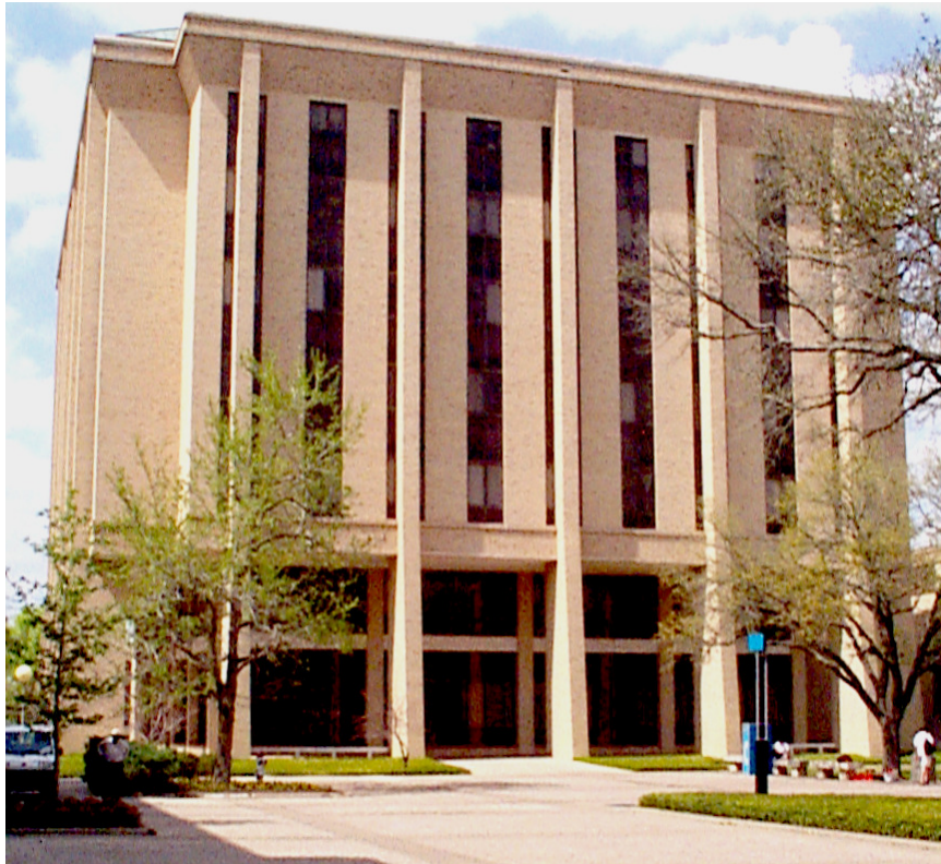
Figure 5-6 Harrington Tower on the Texas A&M main campus [72]
