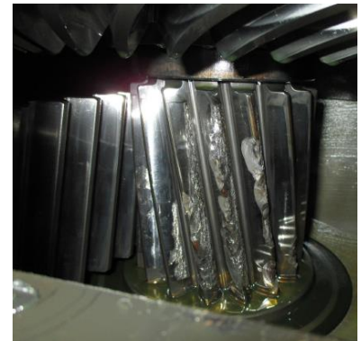
Figure 2. Damaged Pinion Teeth
