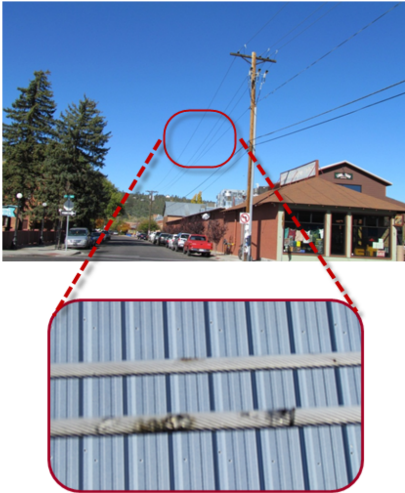
Figure 7.21: Pictures of the location of conductor slap and arced conductors
