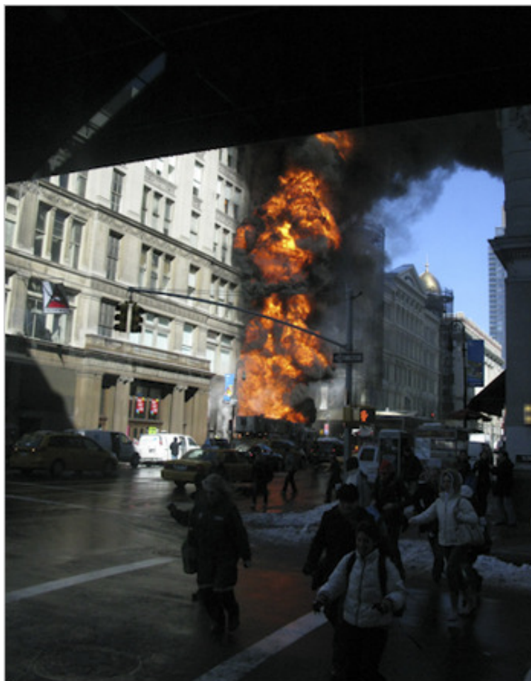
Figure 1: Explosion in a transformer vault, February 11, 2010.
