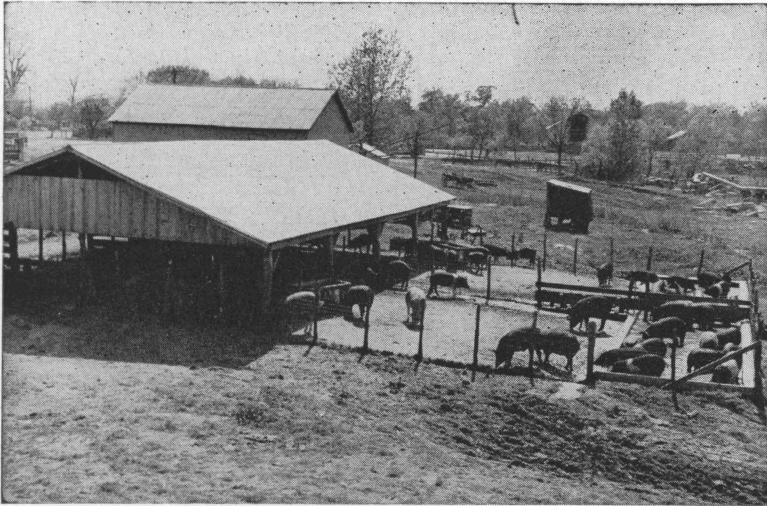
Concrete Feeding Floor with Shed and Wallow
