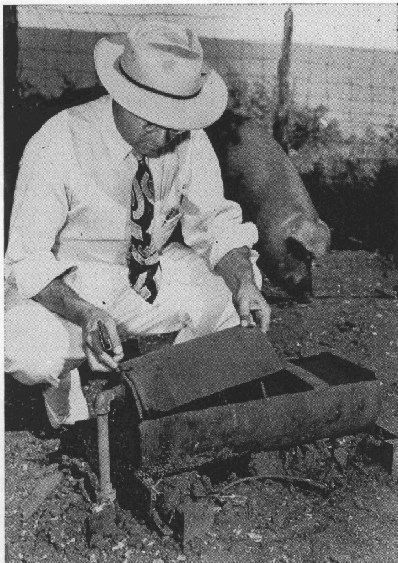
Water Trough Made Out of Oil Field Pipe (Note partition between float-valve and drinking place)
