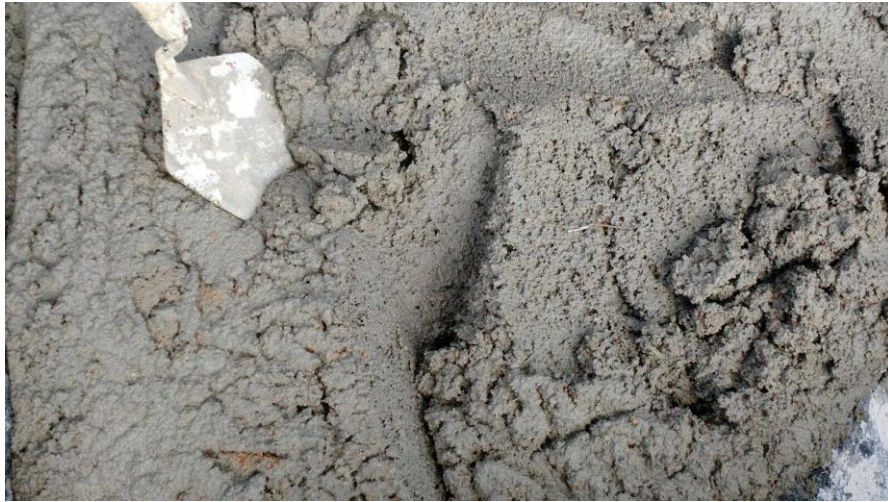
Figure 19: 1:1:6 cement: lime: water mortar mix
