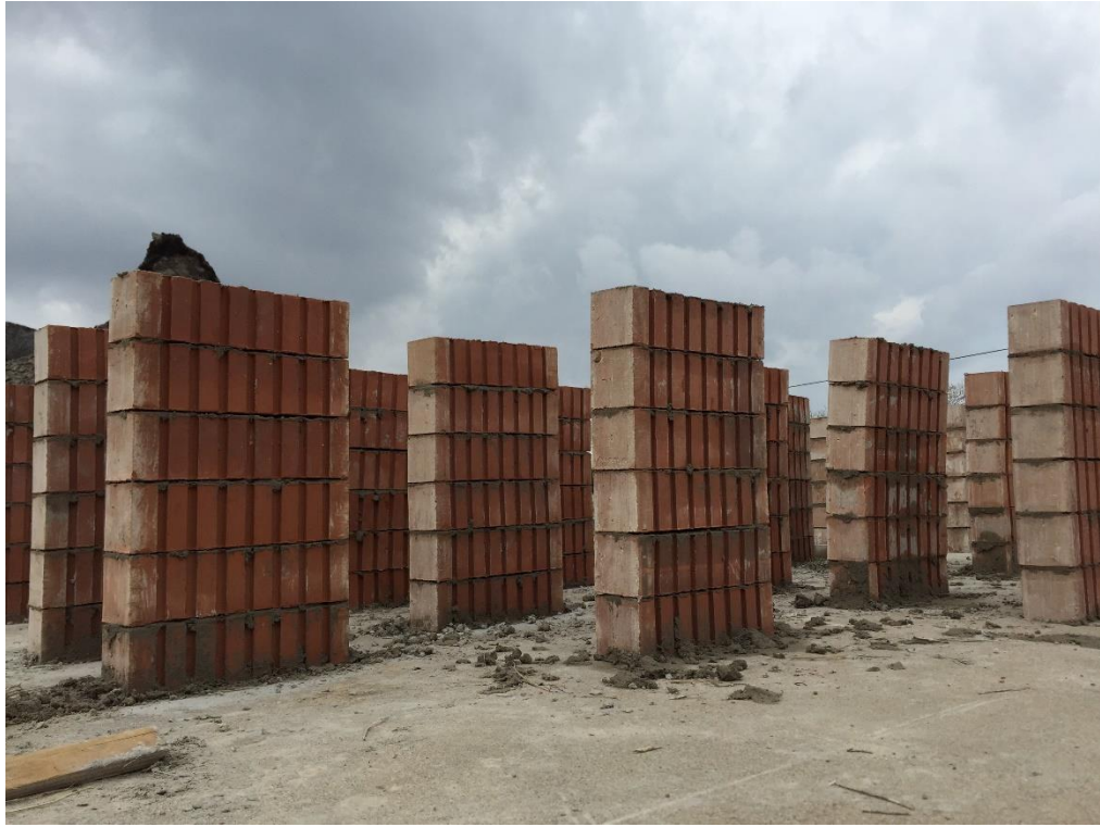
Figure 17: Brick prisms molded out for flexural strength testing
