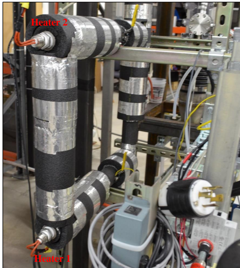
Figure 25. Heating loop (6 kW)
