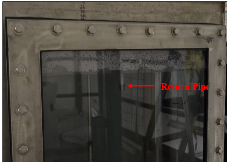
Figure 61. Water level in tank during system cleaning
